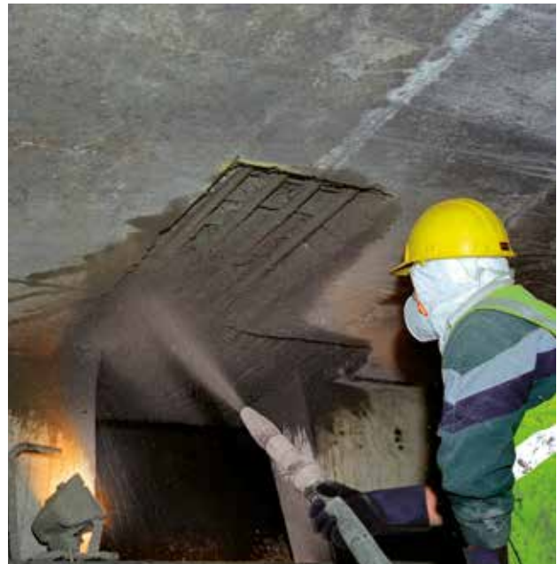
Sprayed mortar
