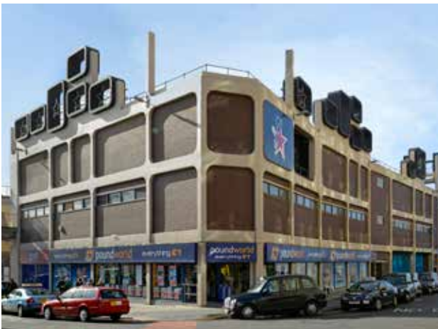
Steel Framed Mansory Buildings
