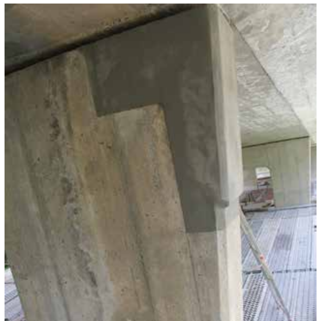
Repair work completed
