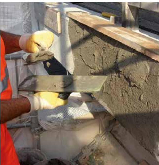
Hand applied mortar
