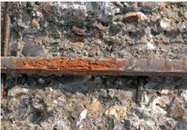
Damage to concrete structure due to insufficient concrete cover and low concrete quality.
