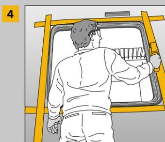
4 ■ If the installation requires a backfilling it is advisable to mask the edge of the flange adjacent to the backfilling with suitable masking tape during this phase
