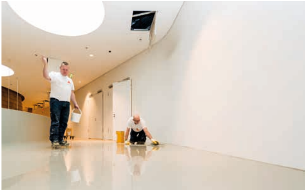
STEP 4. A wide selection of liquid resin products is available in an almost unlimited amount of colors to address many types of use. Decorative flakes or anti-slip aggregates may be broadcasted into the wet surface.
