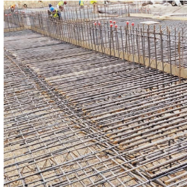
Water treatment plant Albacete, Spain: Sika Waterbar® FB-125
