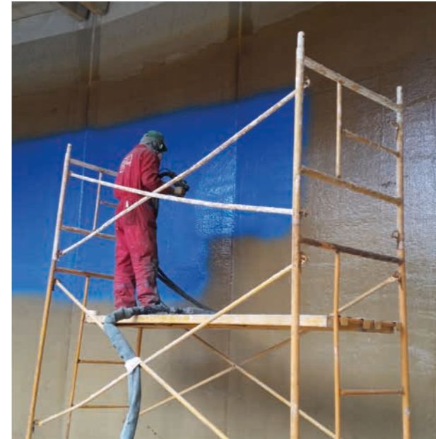
Basin San Esteban, Spain: 800 m 2 of Sikafloor®-161 and Sikalastic®-840 ES.
