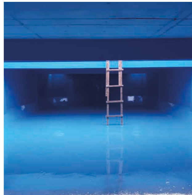
Drinking water tank, Oman: Multi-layer: Sikafloor®-161, Sikagard® PW in blue color.
