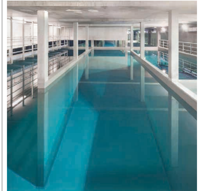
Drinking water treatment plant Kluizen, Belgium: Sikalastic® M 808
