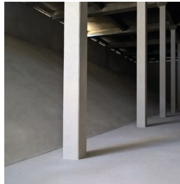
Reservoir Loaysa Granada, Spain: approx. 12'500 m 2 of Sikalastic®-6100 FX.
