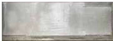
Mortar with good crack behavior.
