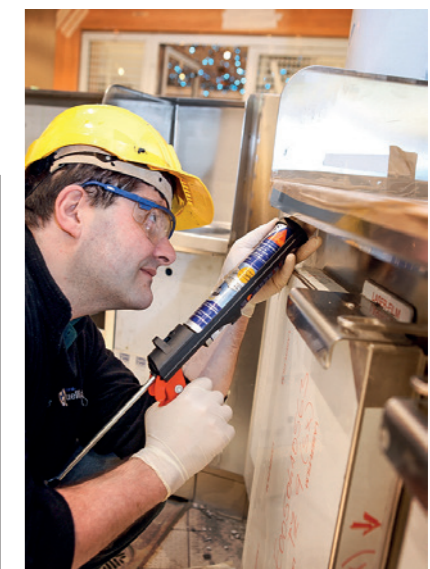
Application of Sikaflex®-591
