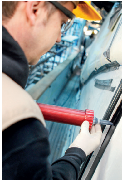
Adhesive is applied to the window frame
