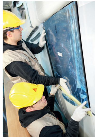
The window is fitted
