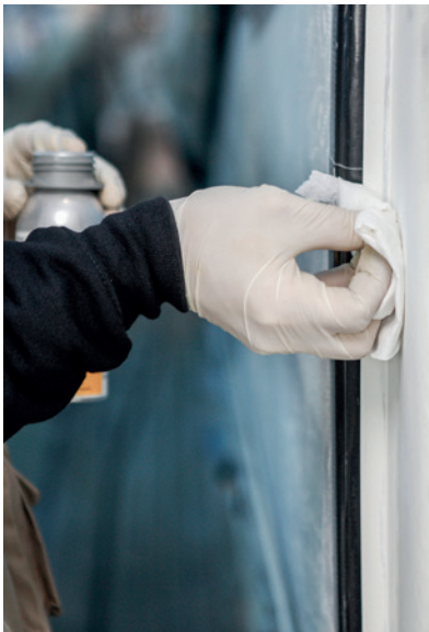
Pre-treatment of the ceramic ink area with Sika® Aktivator-100
