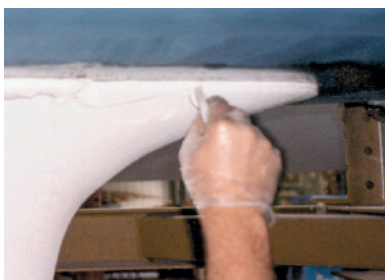
The joint is tooled off and finished
