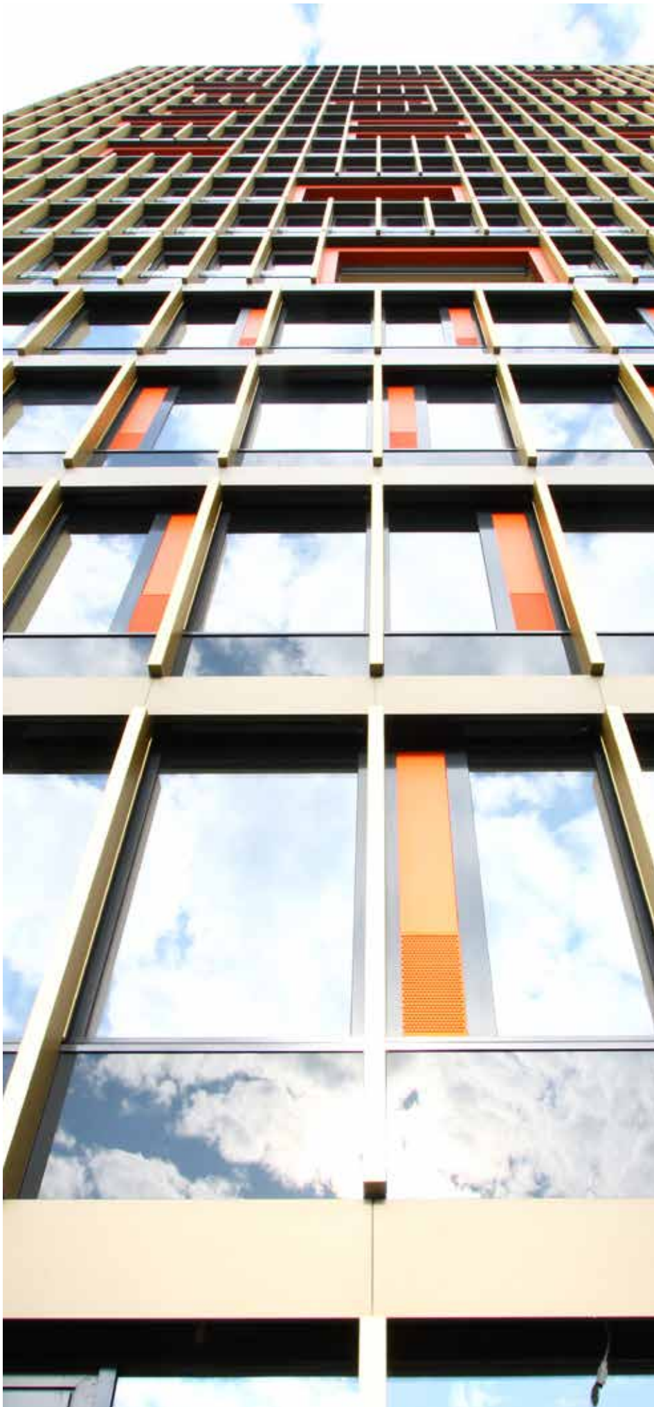
left: Leutschentower, Zurich, Switzerland, 2011 Architect B trix Consolascio; Architekten AG, Zurich Window manufacturer Baumgartner AG Window type Wood/aluminum with opening lights bonded with SikaFast®-5201 NT
