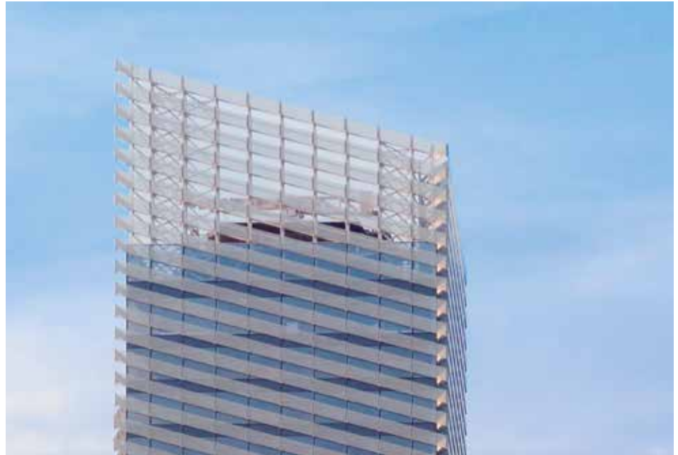
Torre Puig, Barcelona, 2013 Architects Rafael Moneo, Lucho Marcial; Facade Permasteelisa Spain. First European project with Sikasil® SG-550
