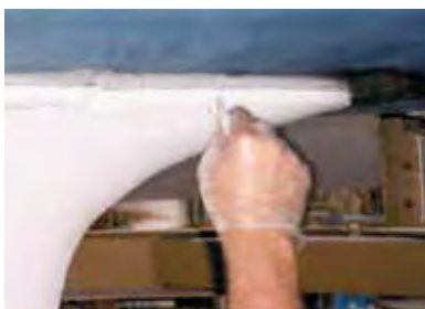
The joint is tooled off and finished
