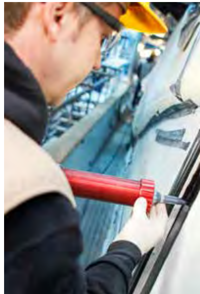
Adhesive is applied to the window frame
