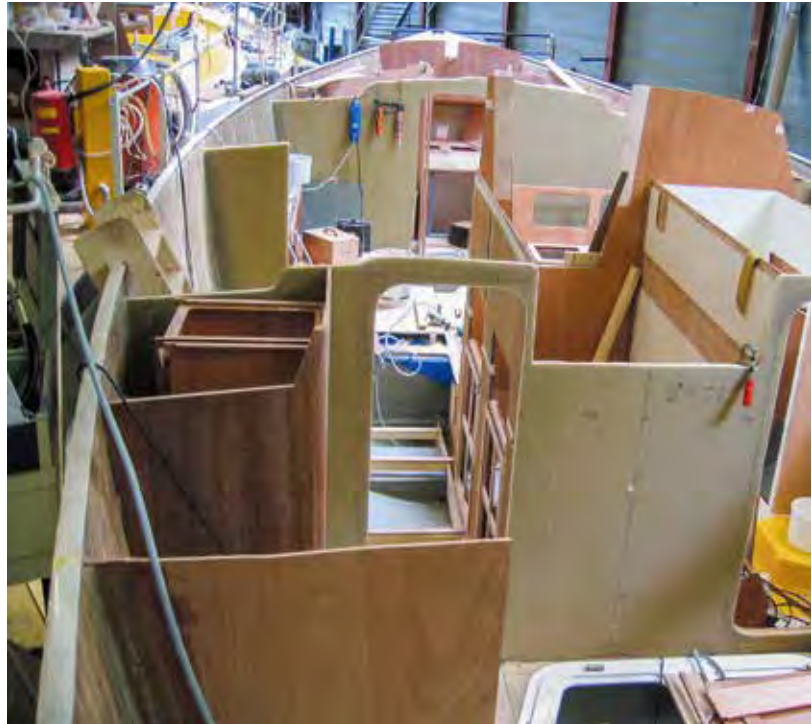
Lightweight panels being fitted to an open hull
