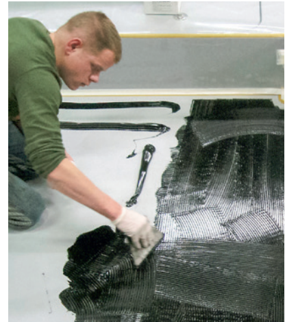
Fig. 44 Application of Sikaflex®-298
