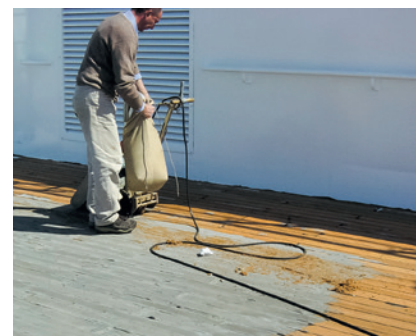
Fig. 13 Sanding the deck
