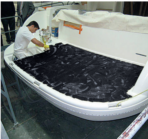
Fig. 19 Application of Sikaflex®-298
