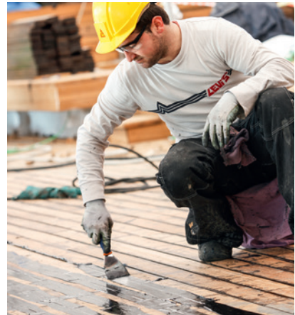
Fig. 12 Compressing Sikaflex®-290 DC PRO with a spatula
