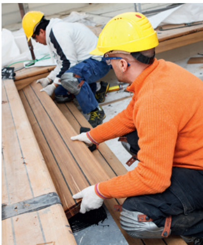
Fig. 4 Putting down the decking
