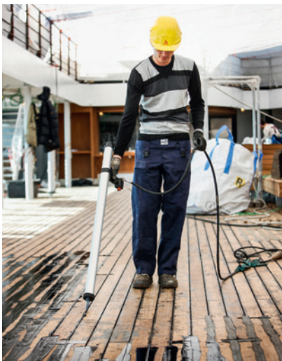
Fig. 10 Applying Sikaflex®-290 DC PRO
