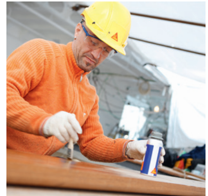
Fig. 8 Carefully applying Sika® Primer-290 DC or Sika® MultiPrimer Marine
